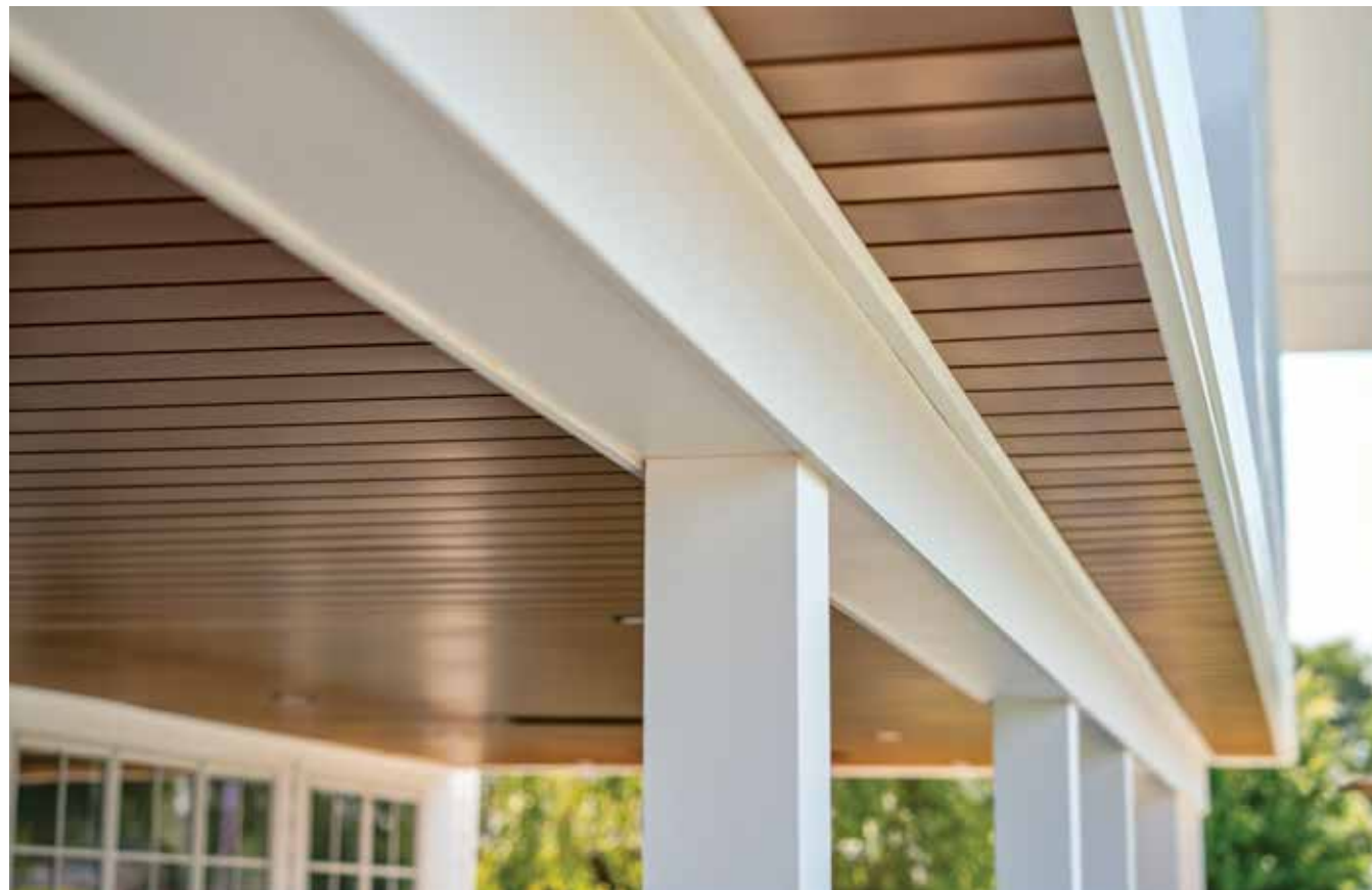
Inside Out® Underdecking in Karri
