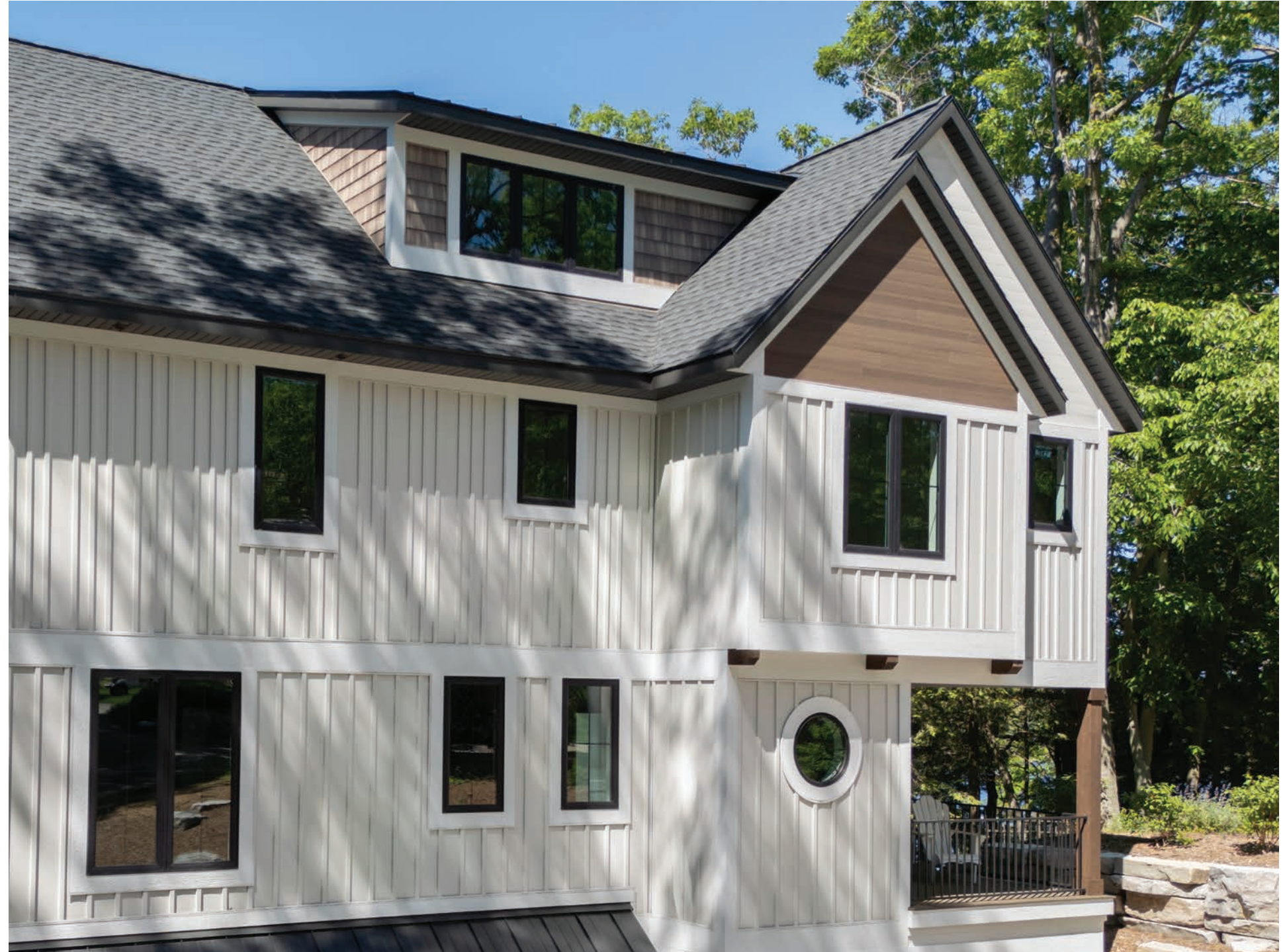
TruCedar 6" & 10" Board & Batten in Fresh Canvas | Vesta 5" Plank in Aged Walnut | Fascia and Soffit in Black, Trim in White
