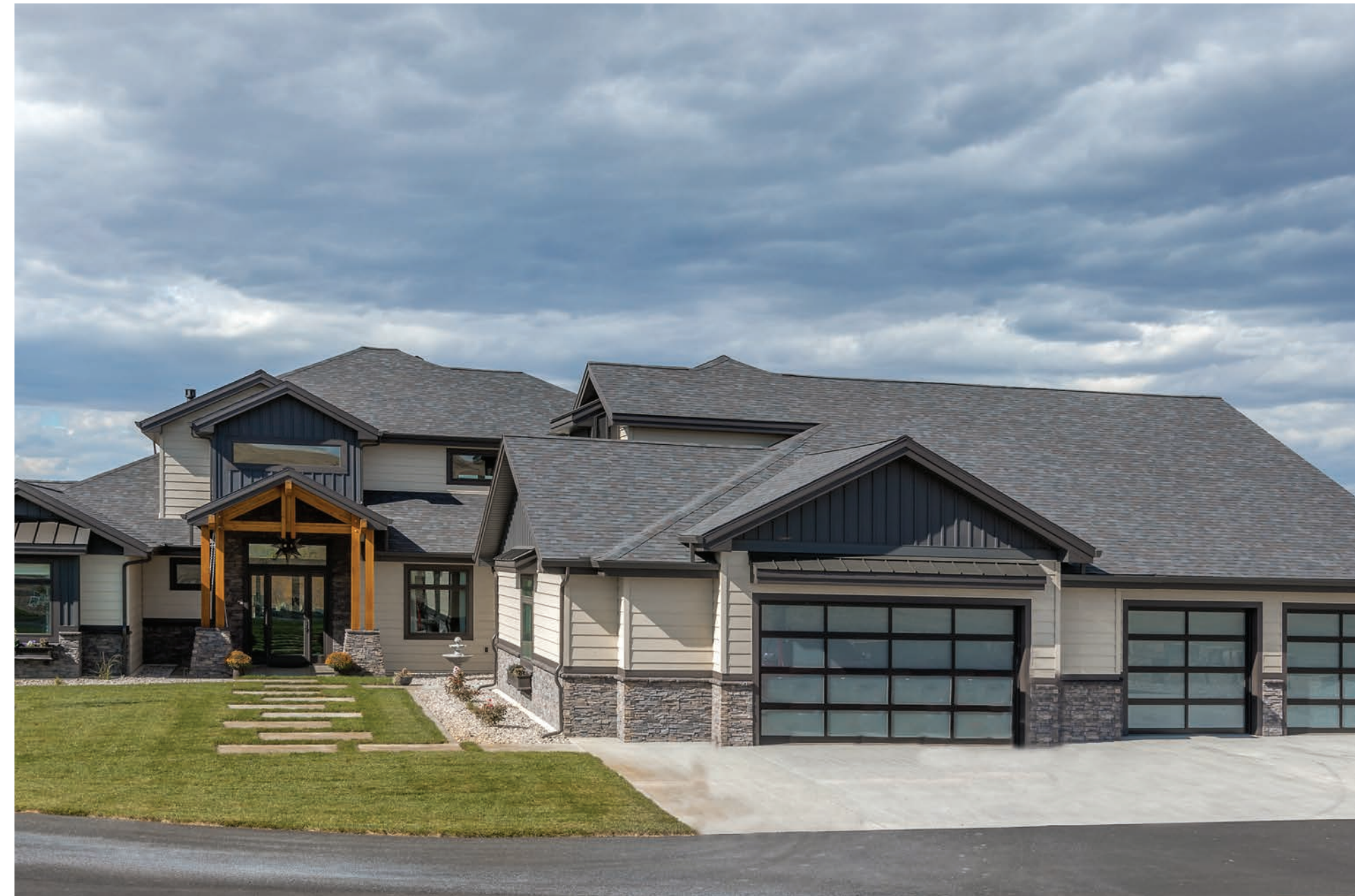
TruCedar Single 8" in Bennington Beige | TruCedar 6" Board & Batten in Ironstone | Drip edge, soffit and trim in Ironstone
