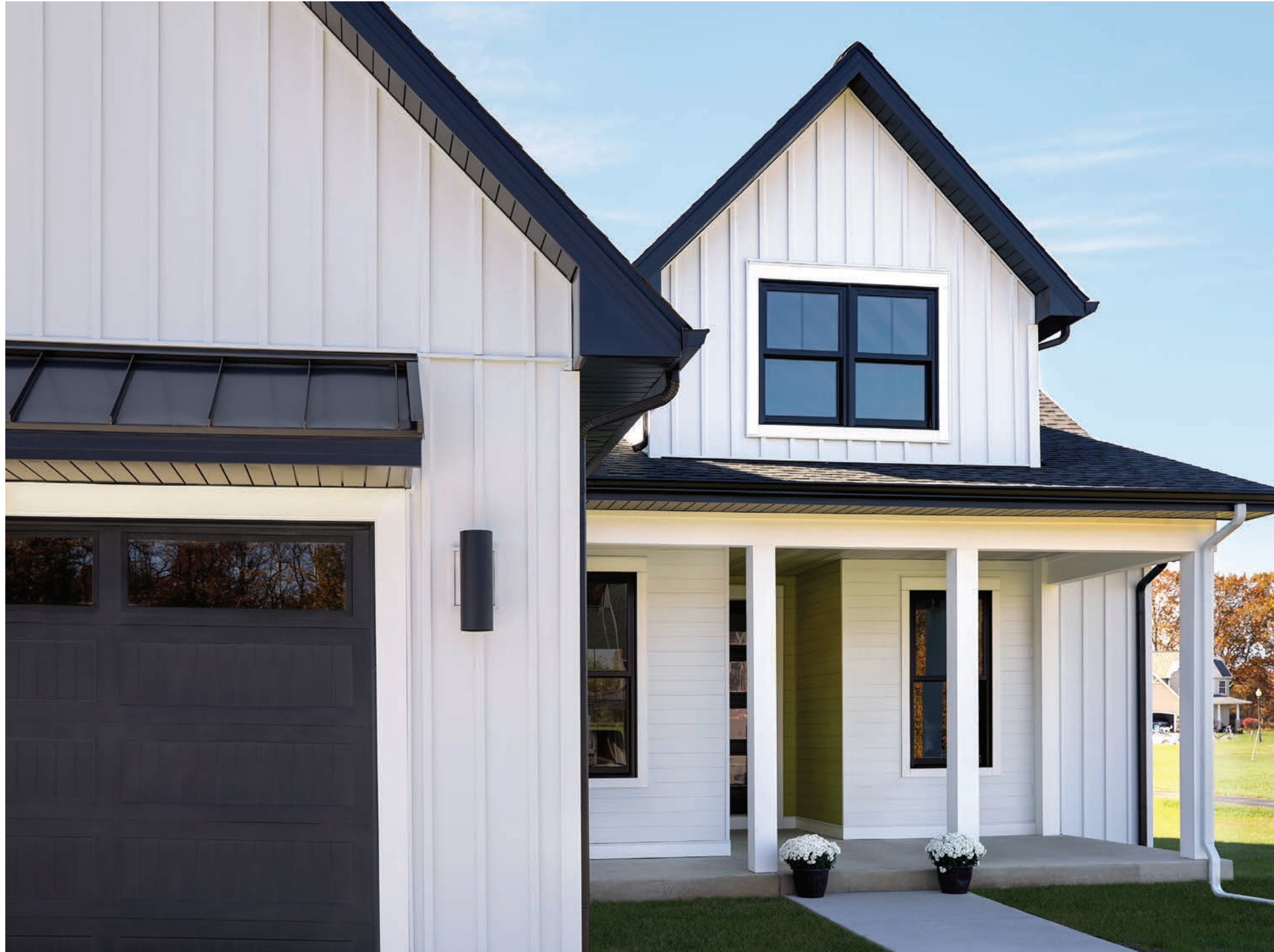
TruCedar in 6" Board & Batten | Vesta Plank in White & Fiddlehead | Fascia, soffit and trim in Black
