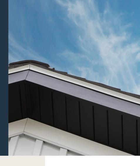
Installers have to be trained to hand notch drip edge in the field. Fish-mouthing can occur when the nose of the drip edge is pinched from incorrect handling.
