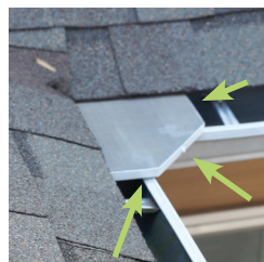
Insert the screen base and screw through the predrilled holes using (3) fascia 1/2" Zip screws.
