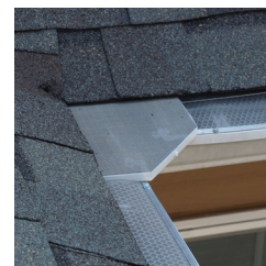
Insert the screen base and screw through the predrilled holes using (3) fascia 1/2" Zip screws.
