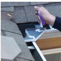
Seal all interior seams on the installed miter.
