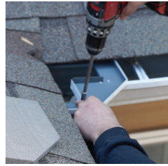
Insert the miter base and place (2) Miter 1/2" Zip screws at the front to secure.
