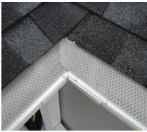
Field Cut Inside Miter (45° Angle)
