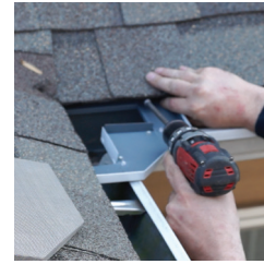
Ensure that the miter base is level and fasten (2) fascia 1 1/2" Zip screws into the pre-drilled holes.
